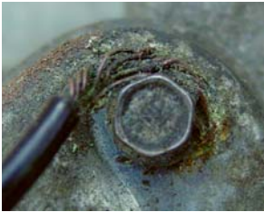
Ground on motor housing as found on my car
