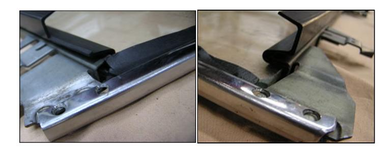
Using an awl or small screwdriver, pry the sash using one frame/sash hole to align the other screw hole between the sash and the frame. Insert that one screw and tighten loosely. Go to the other end of the sash and do the same. Once one screw on each side is installed, use the pry tool to align the next screw and tighten, ensuring the countersink in the frame is centered over the sash threaded hole. Do the same on the remaining end, then tighten all screws securely.
