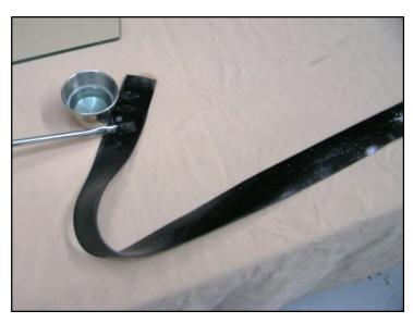
Install the sealing tape into the frame channel so it's even on both sides. Measure and mark the inside corners and cut a notch in each corner for the bends.
