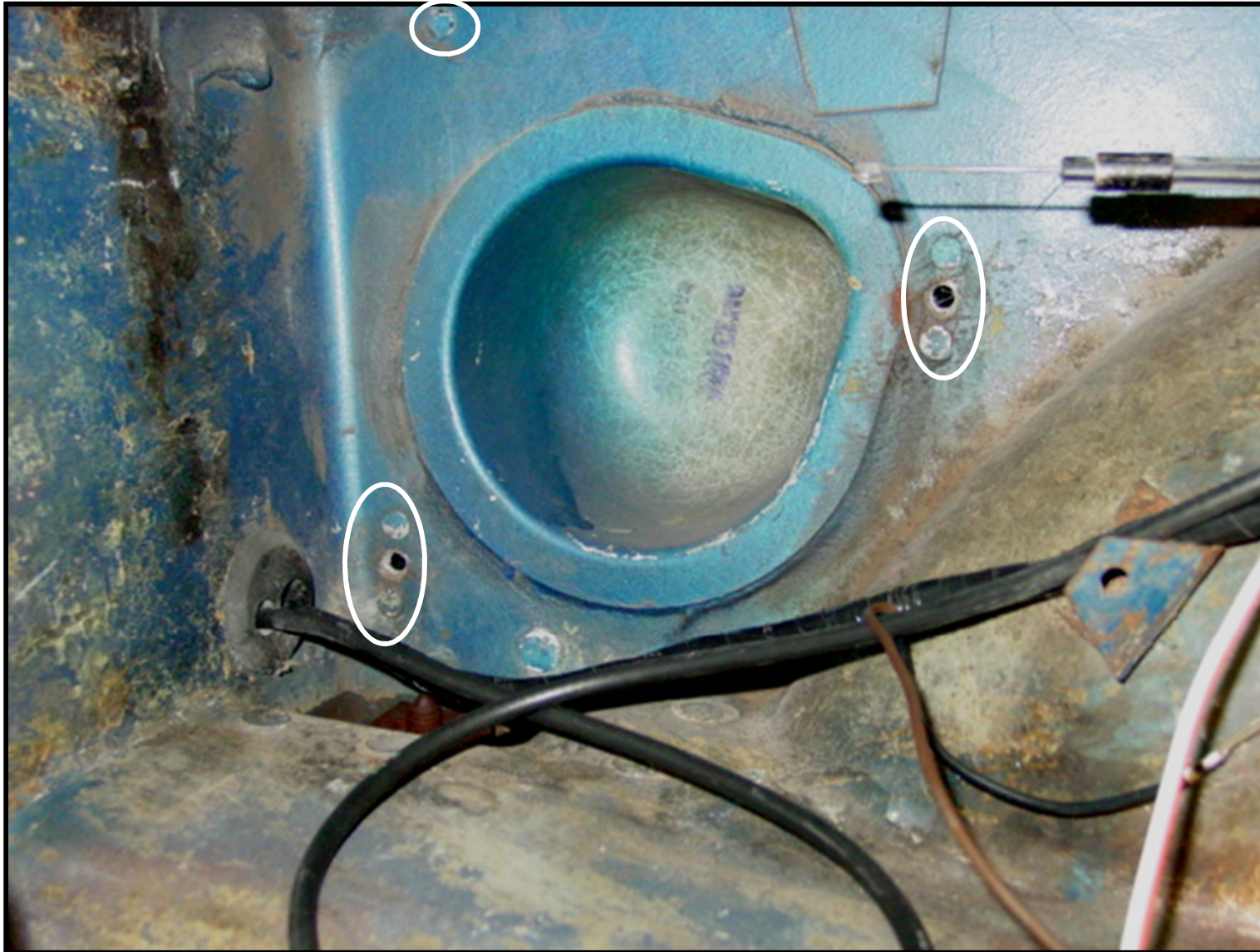
Inside view of the pocket for the blower motor assembly. The nut plates for the mounting bolts are shown in the ovals.
