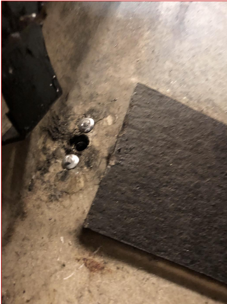
11) Tank Strap Anchor nut repaired
