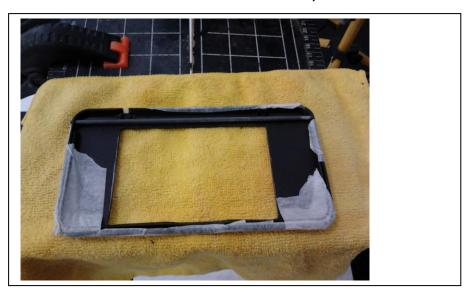
6) With the final hole cut, and top side holes drilled, and rod in place, final fitment of the monitor was made in the hole, just to be sure it was OK.
