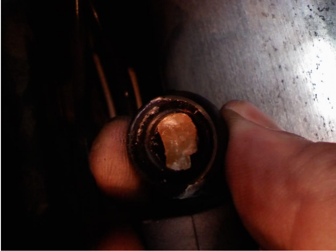
New bushing going in. I used vice grips..
