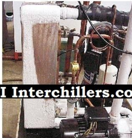
Photo of the same phenomena visualized by ice deposit on outside of the heat exchanger
