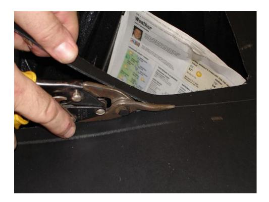
Note: Making a rough cut hole in the shroud first about ½ inch or so inside your scored lines will make it easier to manipulate the plastic when making the finish cut.
